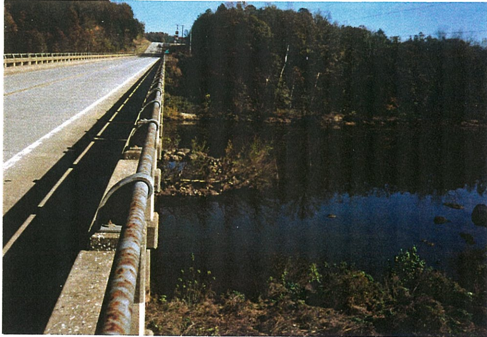
Photo 1: View facing east along downstream face.
