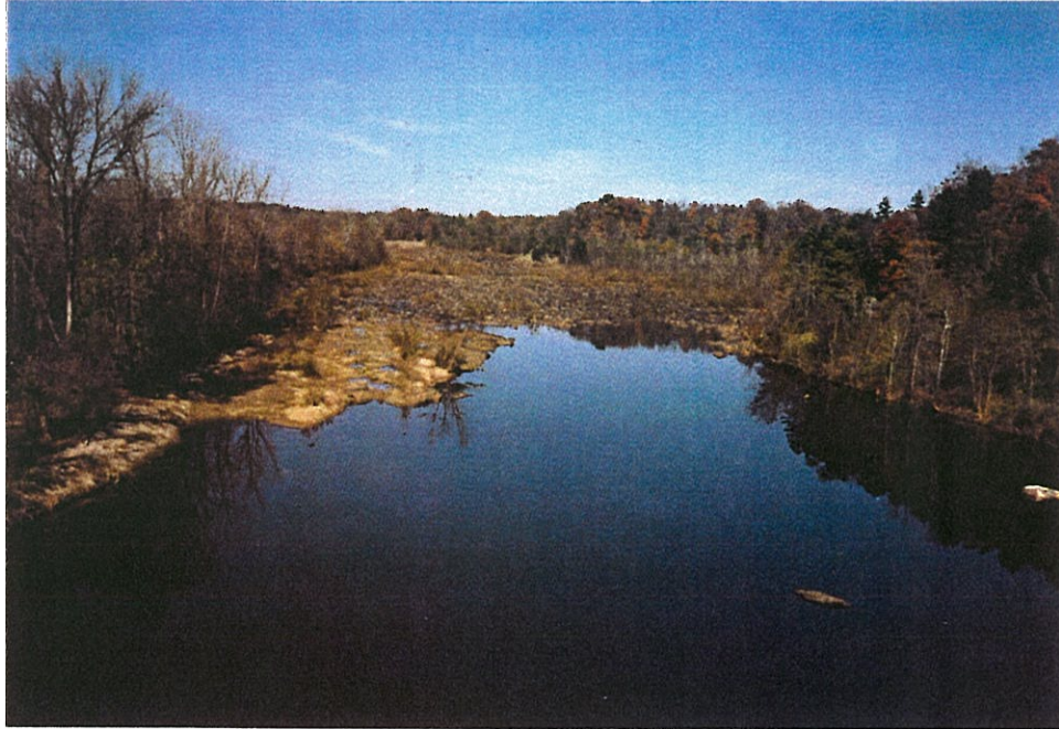
Photo 3: Upstream view, note weir (extreme center left).
