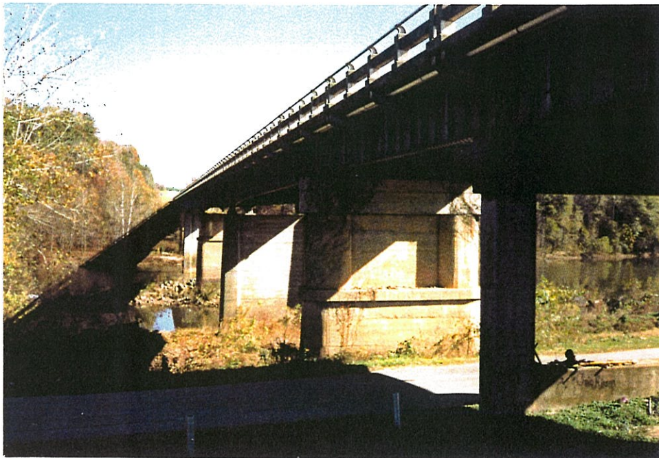
Photo 12: Eastern view of upstream face. Pier 2 is in right foreground followed by A, B, C, and D.
