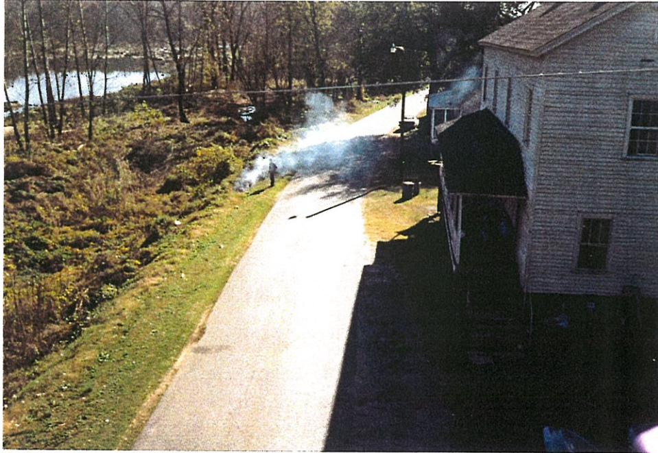
Photo 9: Downstream view at west overbank from bridge.
