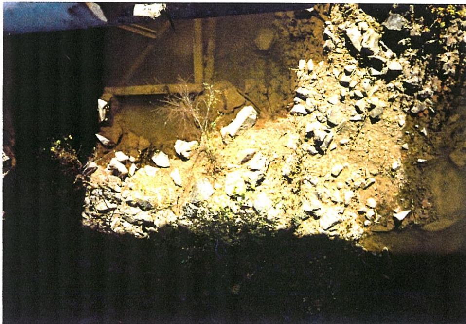
Photo 8: Downward view of coffer dam island around pier "C".
