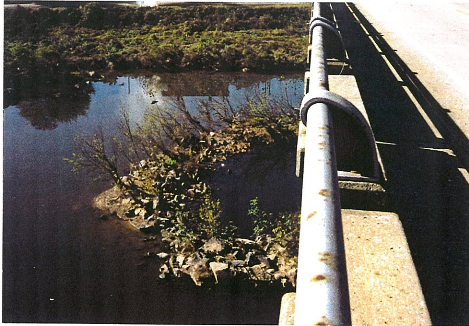
Photo 7: Western view at coffer dam island around pier "C".
